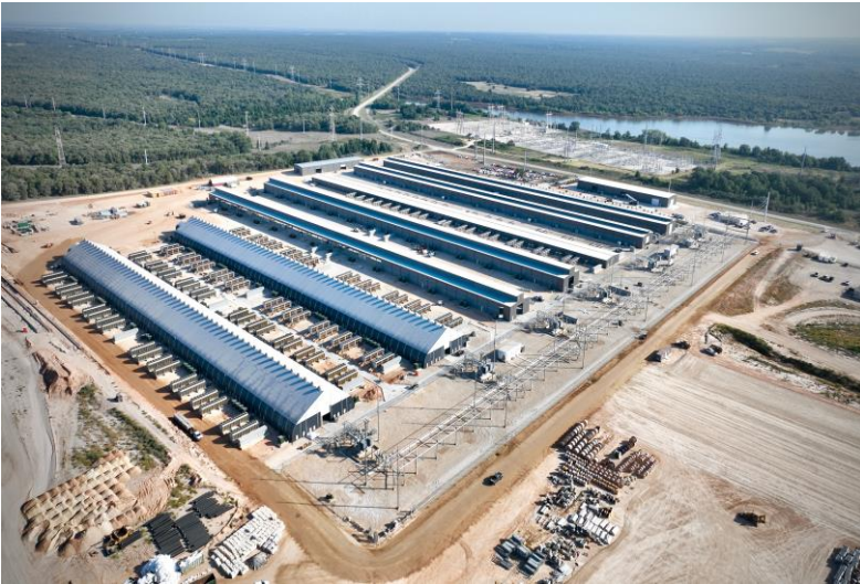
The Present (2022) – 600MW Permanent Structure Data Center – Rockdale, TX
