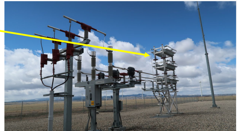
Shunt Capacitor Bank at POI
