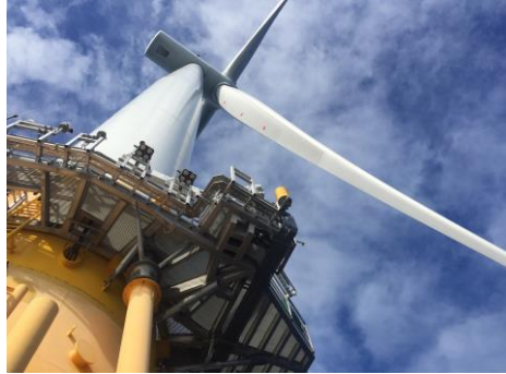
Photo: Equinor Scotland 30 MW 5 Turbines – Credit: Walt Musial
