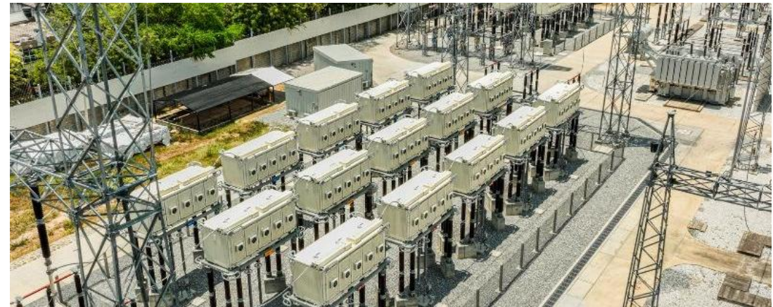
SmartValve Installation – ISA TRANSELCA, Colombia
